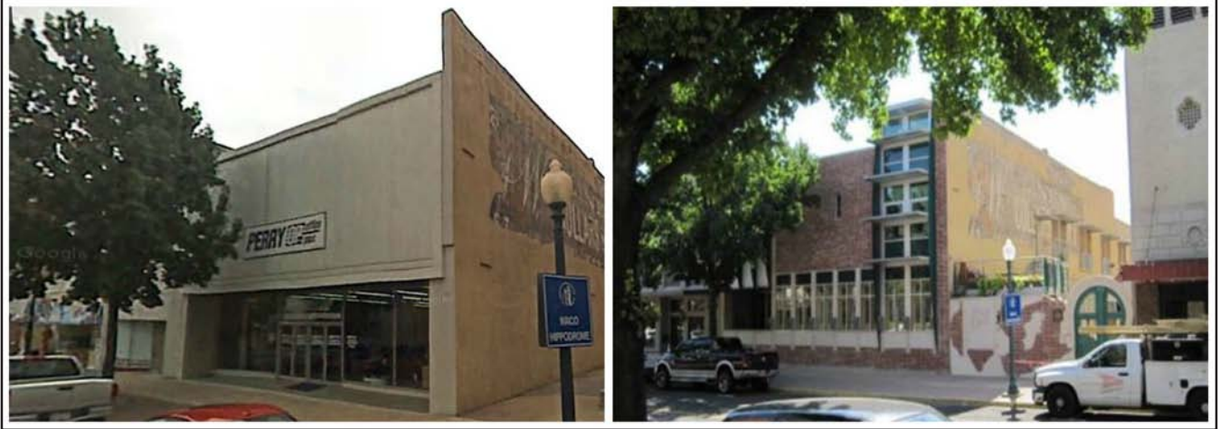
Figure 4.5–4.6. An example of rehabilitation of a remaining historic building.
