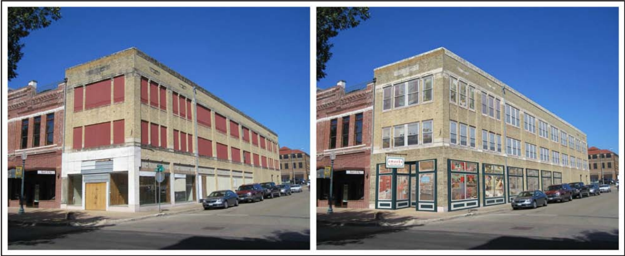
Figure 4.9–4.10. Upper floor windows covered (left) and Main Street design staff suggestion for new storefront and revealing upper floor windows (right).
