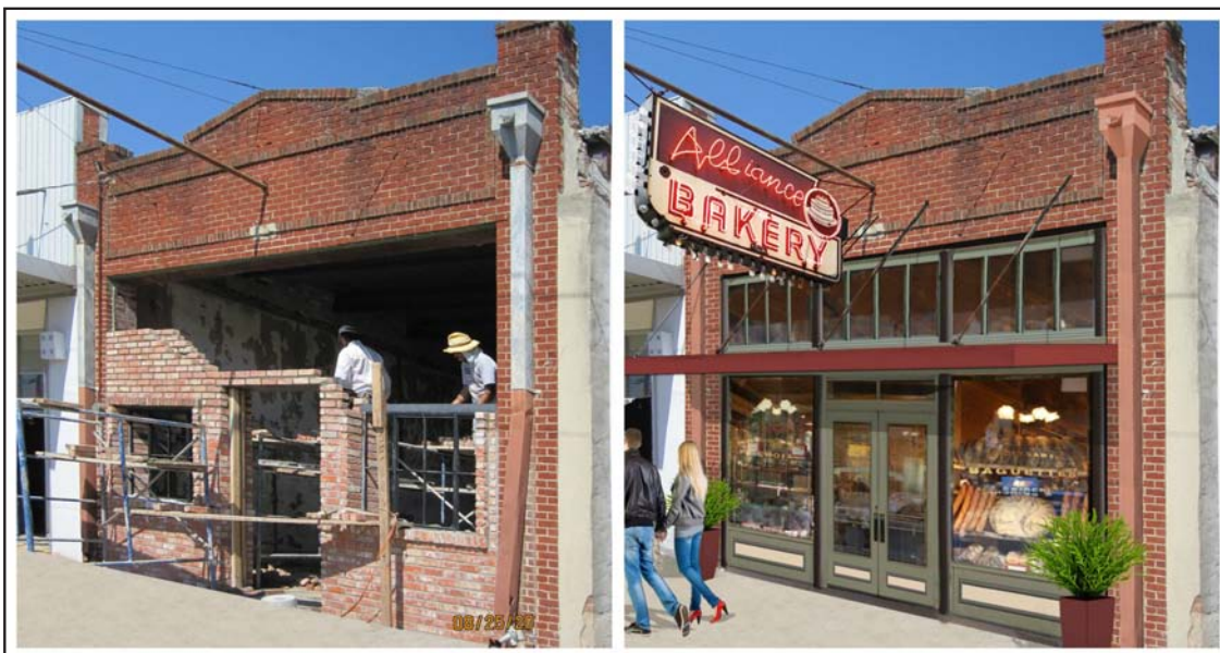
Figure 4.7–4.8. Facade under construction (left) and Main Street design staff suggestion (right).
