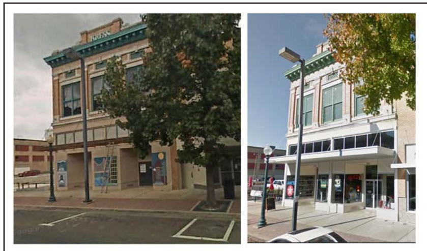
Figure 4.3. Kress Building Facade.
