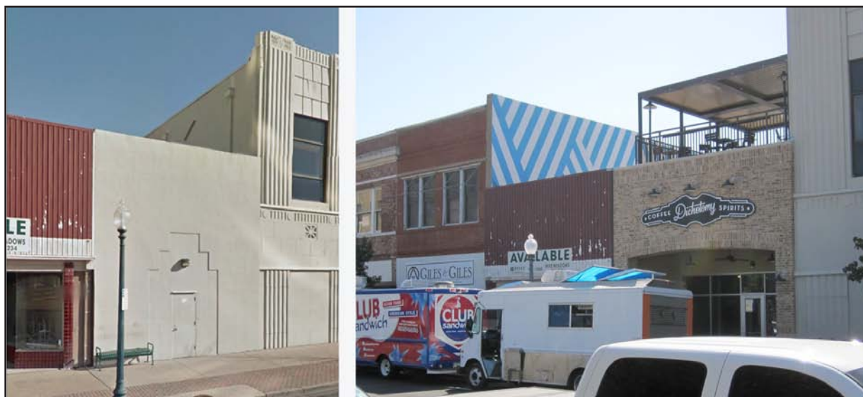
Figure 4.4. A completed facade on an under-utilized building on Austin Ave.
